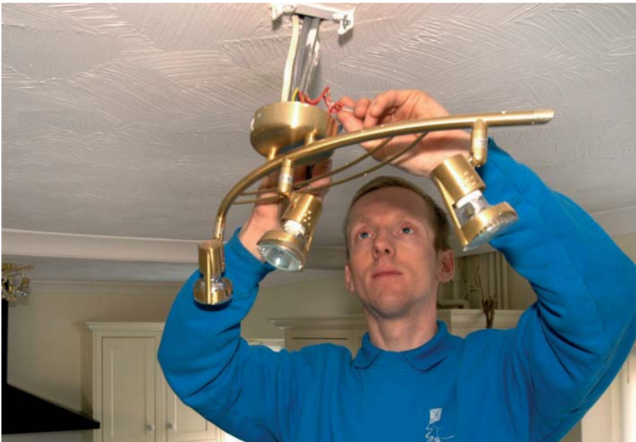
Replacing a light fitting does not require approval
