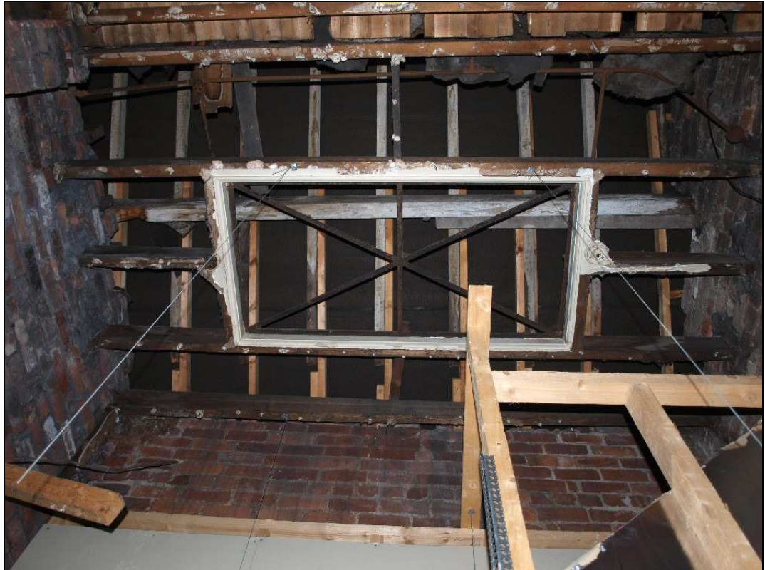
Figure 15: Detail of former ceiling construction
