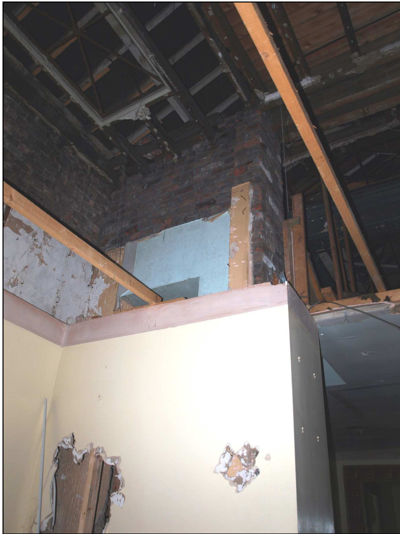
Figure 12: Internal wall stub
